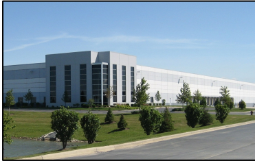
Navistar Joliet, Illinois Leased 522,500 s.f. vacant building and expanded it by over 50% to 860,100 s.f.
