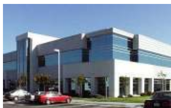
Trion Worlds 1200 Bridge Parkway 52,000 sf
